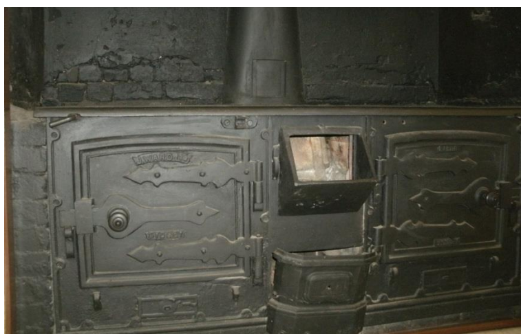
The renovated range at the Binnaway Railway Barracks (2018)
