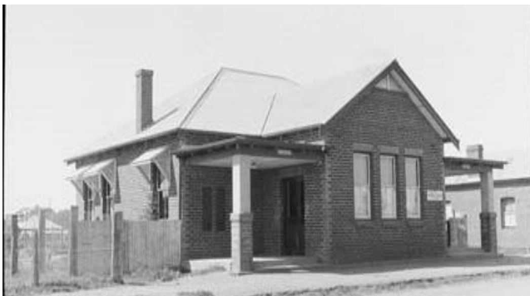
Binnaway Post Office – built 1939-1945 (National Archives)
