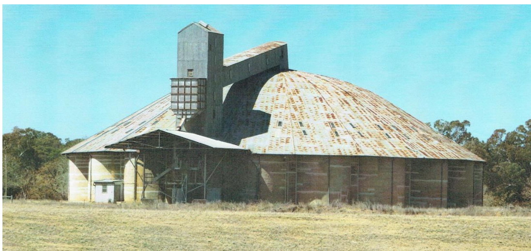
Concrete Silo – Baradine
